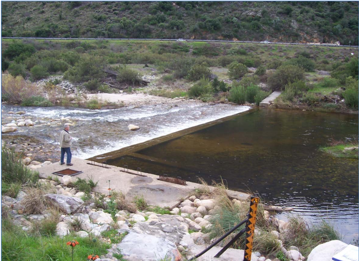
Figure 11: The Proposed Location for the BBTS Diversion Weir
