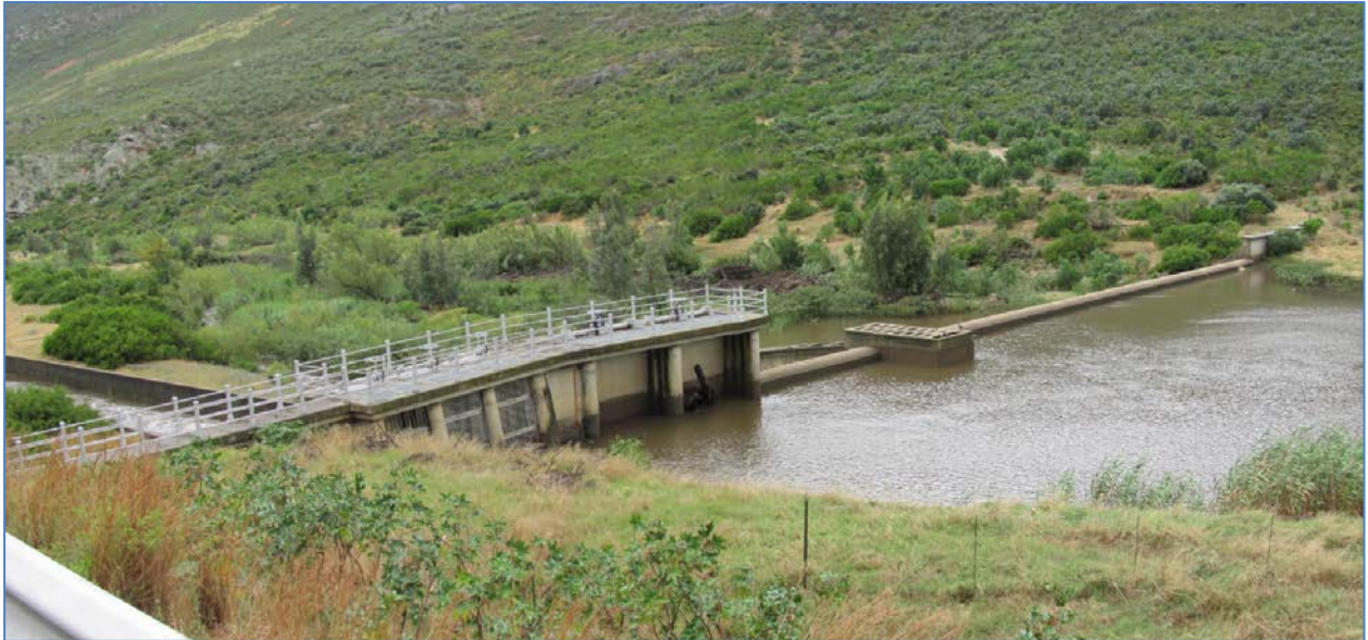
Figure 4: The Existing Klein Berg Diversion Weir
