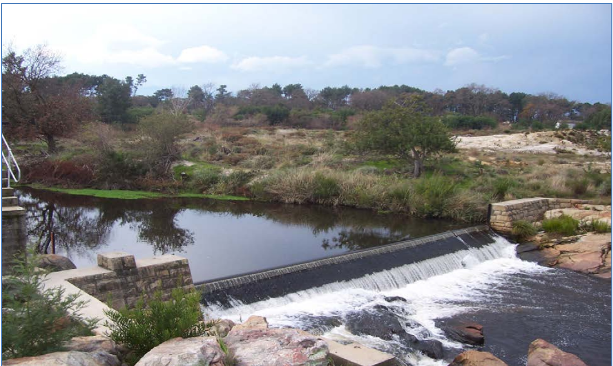
Figure 15: The Existing Stream Flow Gauging Station, H1H003 at Ceres Golf Club
