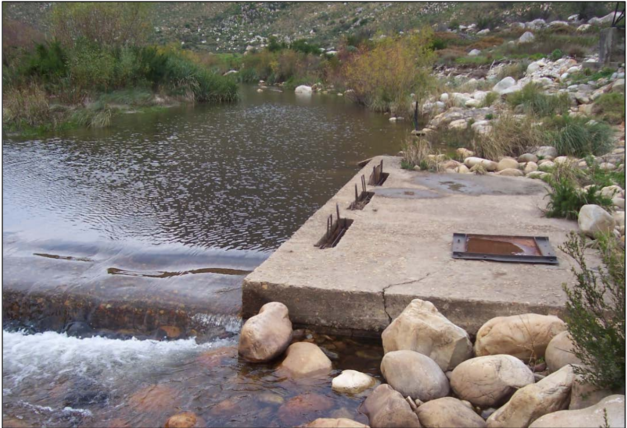
Figure 14: The Existing Artois Canal Intake Structure at the DWA Flow Gauging Station (H1H006)
