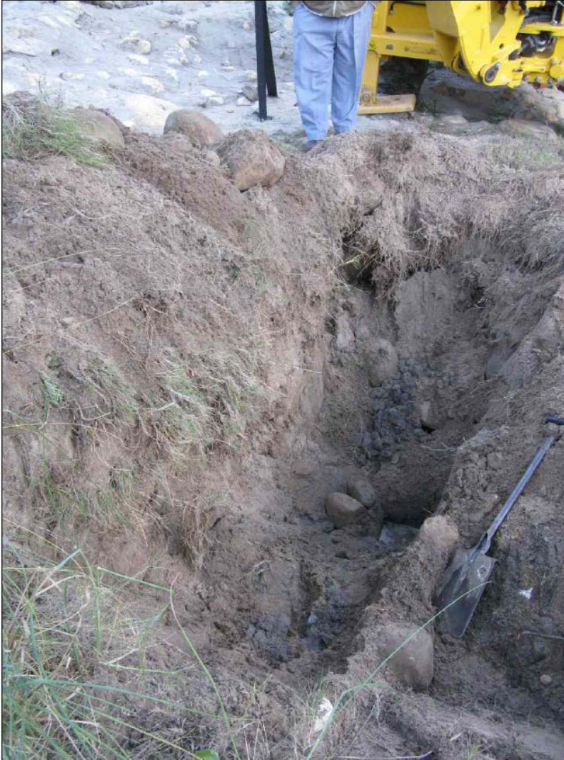
Figure 49: Trial Pit Excavation Showing Alluvial Conditions at the Weir Site
