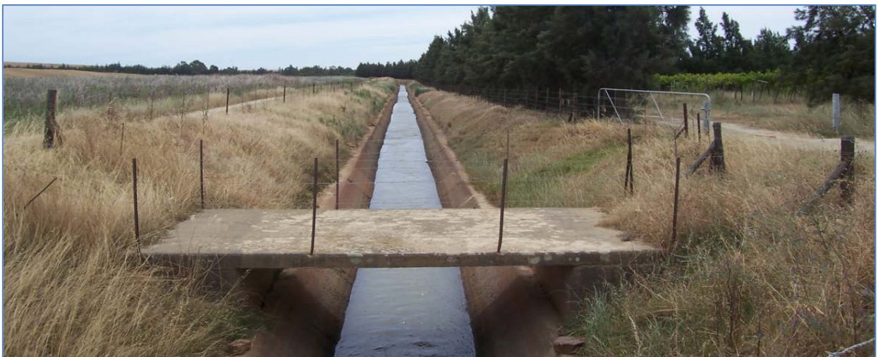
Figure 5: The Existing Voëlvlei Dam Outlet Canal to the Berg River
